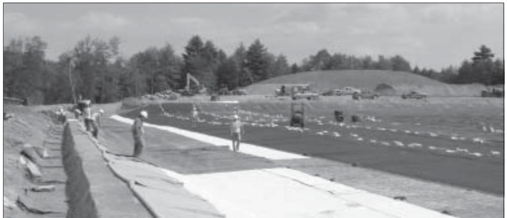
Liner crews install HDPE geomembrane in the secure landfill cell.
