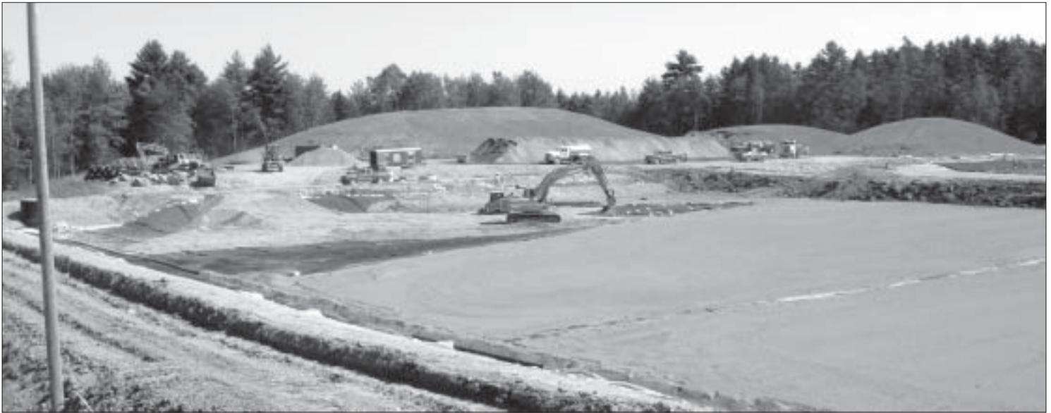
Sargent crews place sand layer and sump stone at the SAPPI secure landfill.
