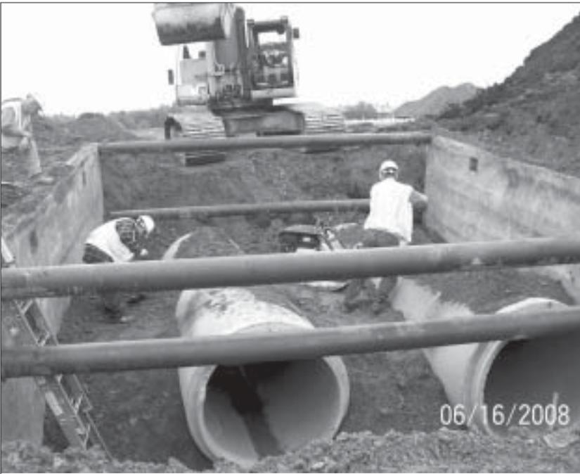
*Twin 48" RC culvert pipes were installed across the runway.*
