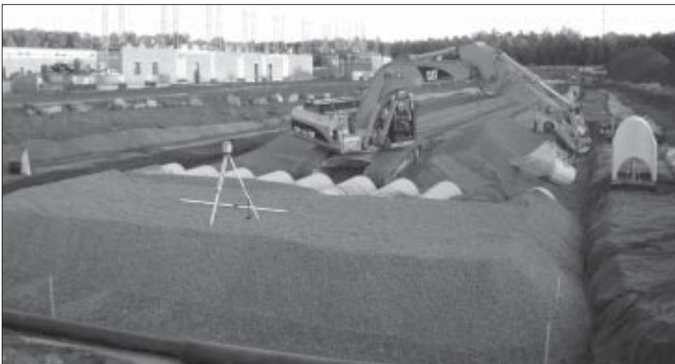
Crews install the underground StormTech system, which will treat stormwater before it leaves the site.
