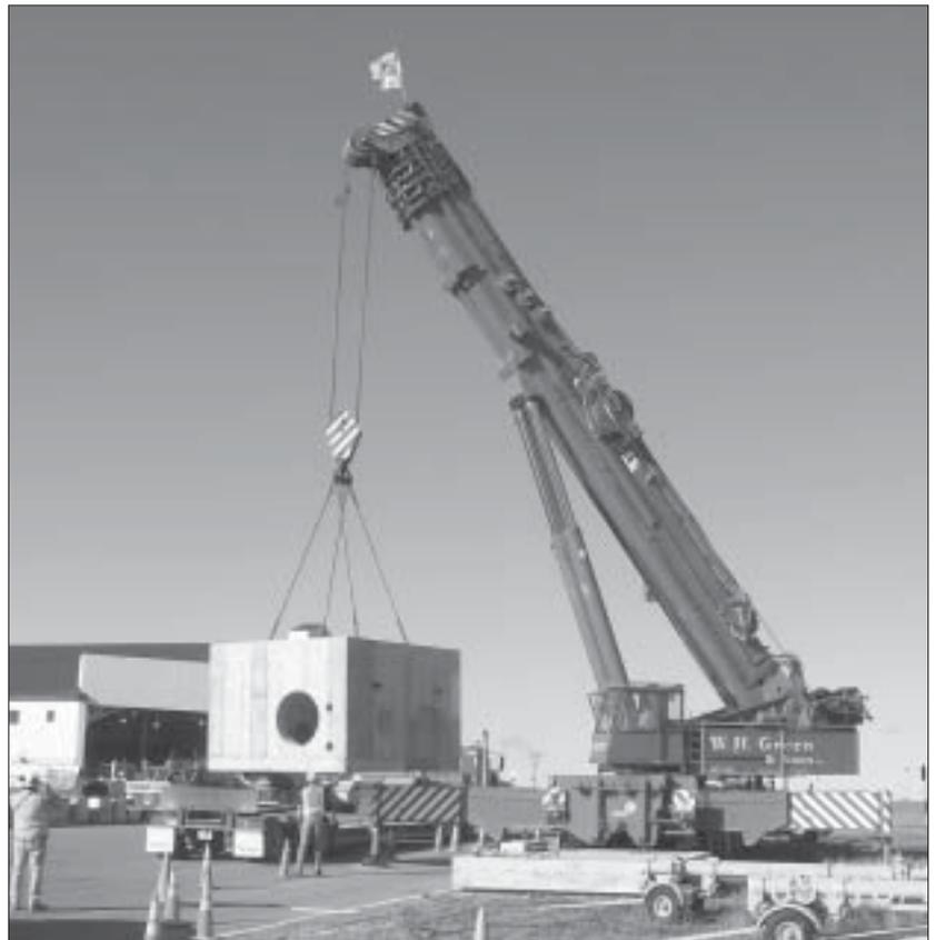
*A 450-ton crane picks one of the DV structures from the lowbed and prepares to put it into position.*
