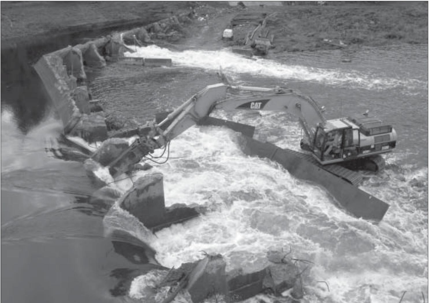
*Greg DeNicola works from behind a wall of steel plates to enlarge the hole in the Ft. Halifax Dam and reduce the water level.*
