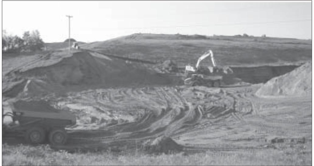
*Sargent crew excavates a future cell to grade for borrow materials in the phase 9-14 section of Waste Management's Rochester, NH, landfill.*
