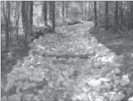
Stream enhancement riprap now protects an old, eroded streambed leading to Penjajawoc Stream.
