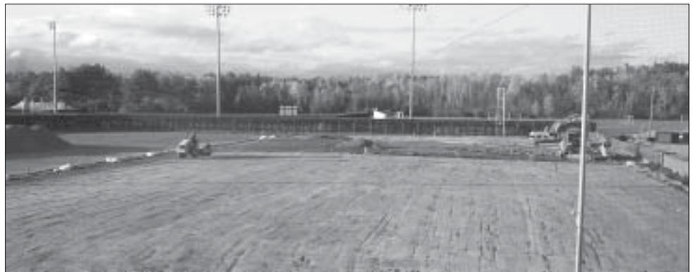
*Sargent crews prepare the subgrade with the underdrain installed at Mahaney Diamond.*
