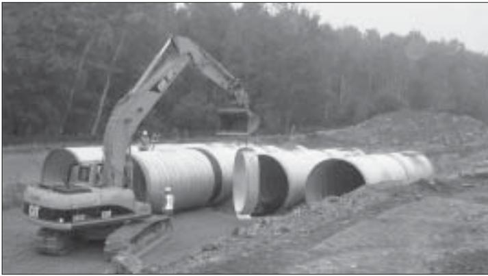
Jake Harris's crew installs the 10' corrugated metal pipe (CMP) stormwater detention system at Bangor Wal\*Mart.
