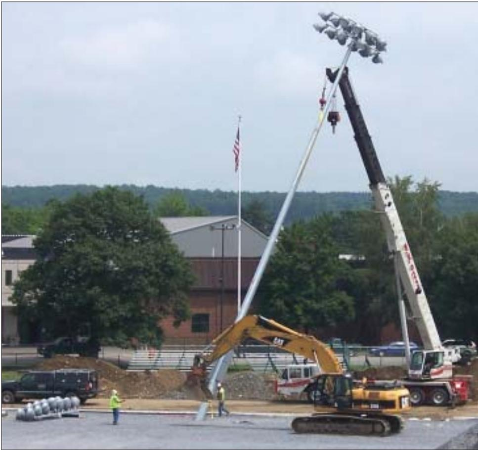
Subcontractor crews lift one of the pro-style lighting fixtures for the athletic field. The fixtures are 80-100 feet tall and are visible from I-95.
