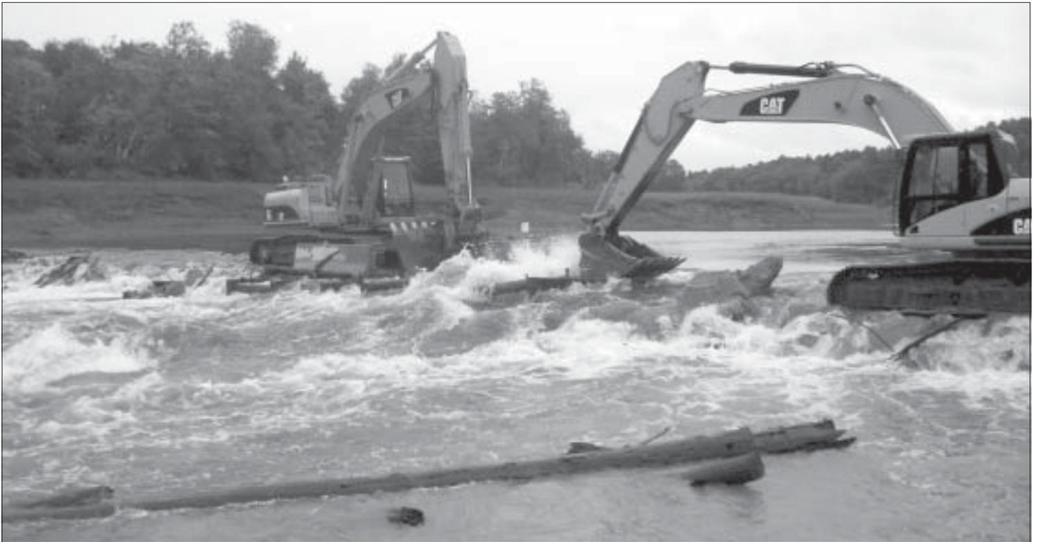
*Operators Steve Renaud and Greg DeNicola place trench boxes in the Sebacook River to allow trucks to use an access road to haul riprap to reinforce the north slope along Dallaire Street. The access road was originally constructed to provide access for a sewer project.*
