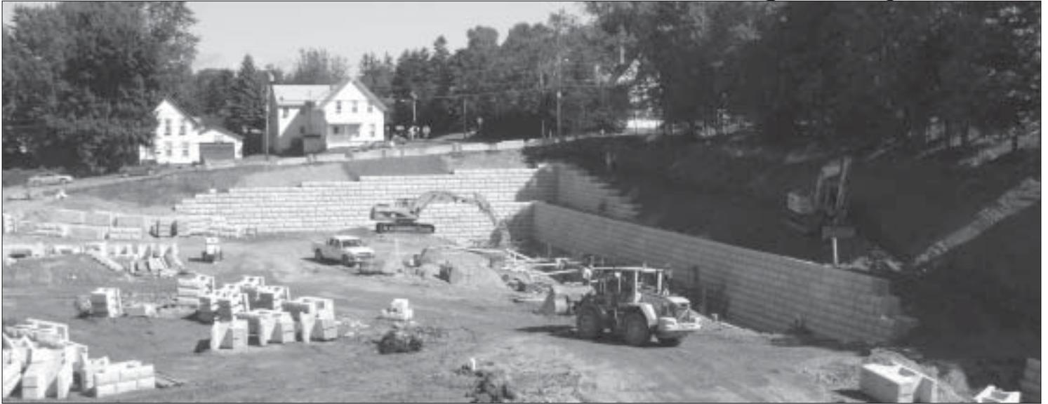
*Sargent crews construct the terraced retaining wall, which had to be constructed in an extremely tight area.*
