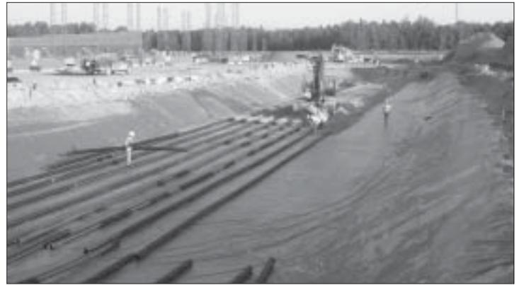
Curt Van Aken's crew installs the underdrain system for the StormTech stormwater treatment system.
