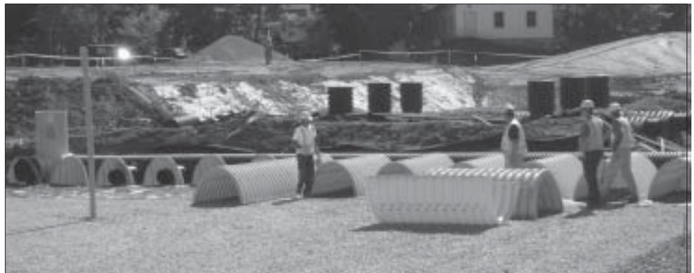
*Sargent crews install the underground StormTech system.*
