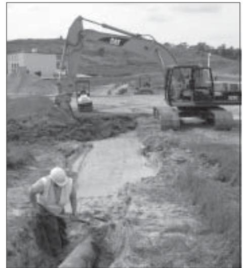
*A Sargent excavator places topsoil over the compacted sand backfill covering the gas main.*
