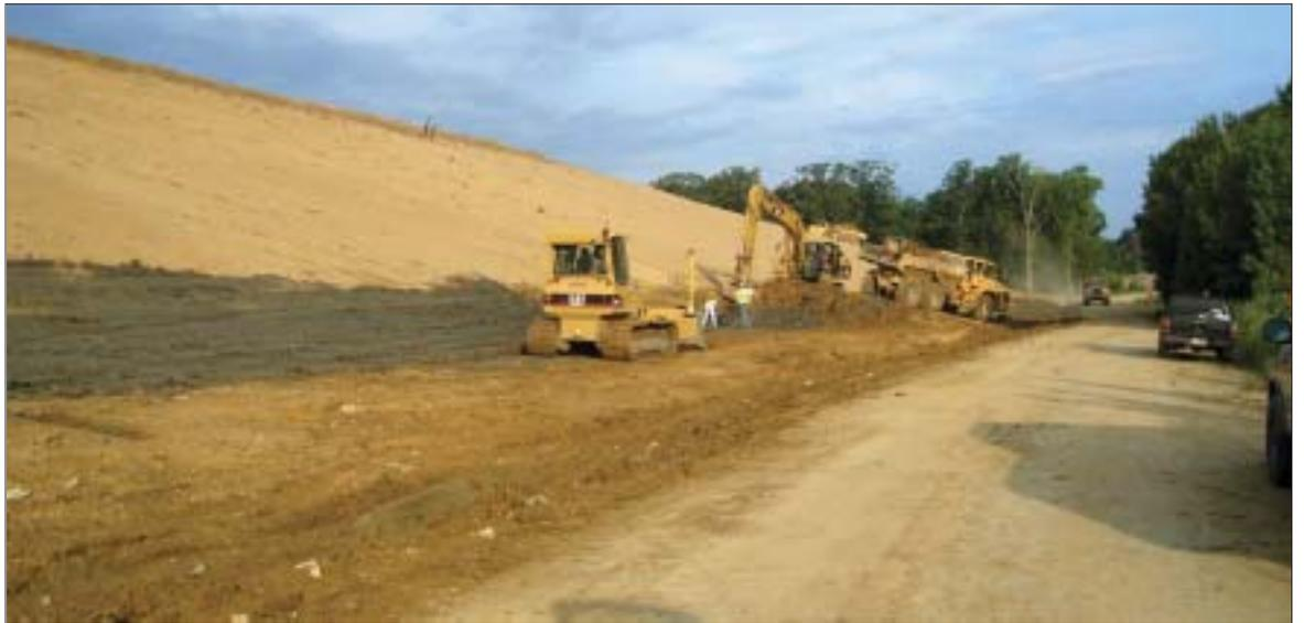
Sargent Corporation crew works on placing a clay plug at the toe of the slope. Operators are Antonio Griffin, Cat D5 dozer; and Tim Cole, Cat 325 dozer. Foremen are Art Robinson and Luther McBee.
