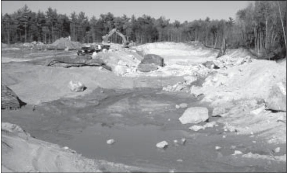
*Steve Renaud operates the Komatsu 600 to make a cut from a future mitigated wetland area and an adjacent pond. A total of 115,000 yards of material is to be removed from this area and placed in the Wal-Mart parking lot and the adjacent Lowe's site. Blasting crews from Maine Drilling and Blasting follow where ledge is found.*
