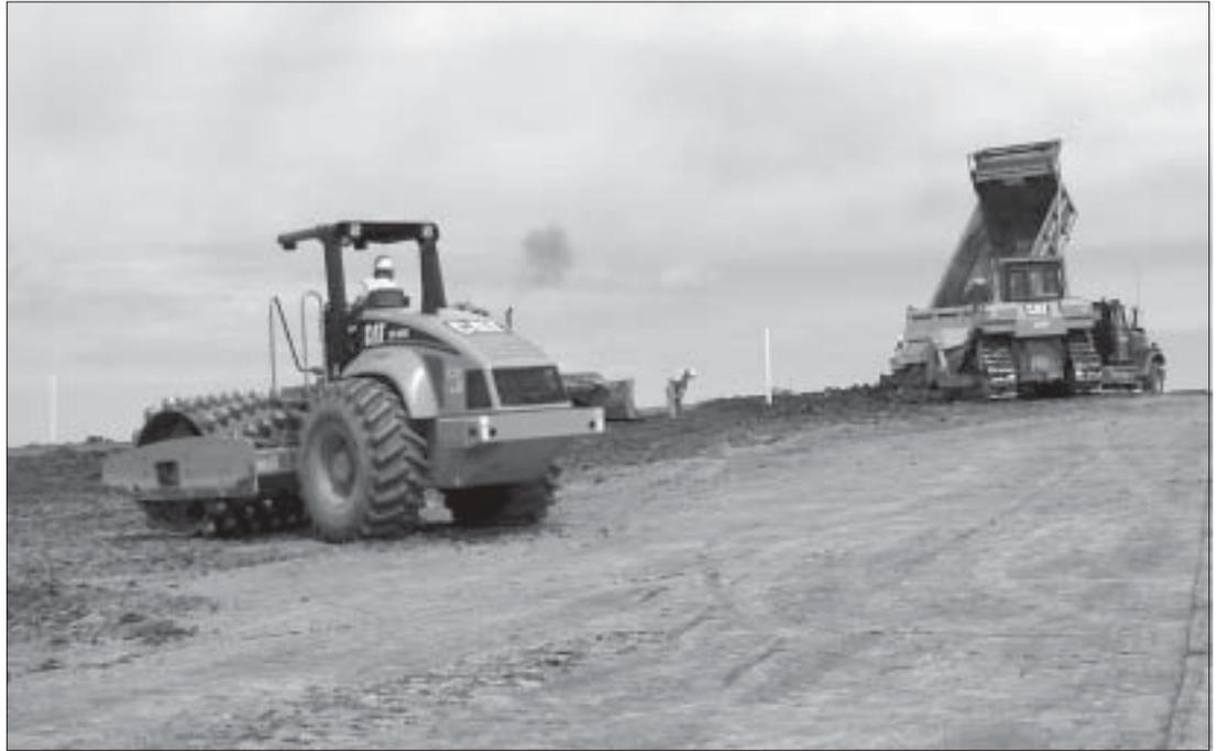
*Ronnie Hall uses a sheep's foot roller to knead lifts of clay together for the cap on a 4-acre section of the Verso landfill in Bucksport, as foreman Jake Harris watches a load of clay being delivered.*
