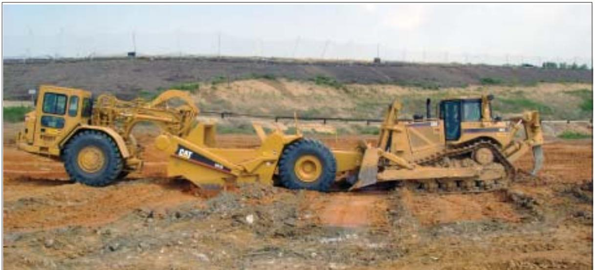
*A Cat 621G scraper is pushed through the cut by a Cat D8T during the excavation to stockpile operations.*
