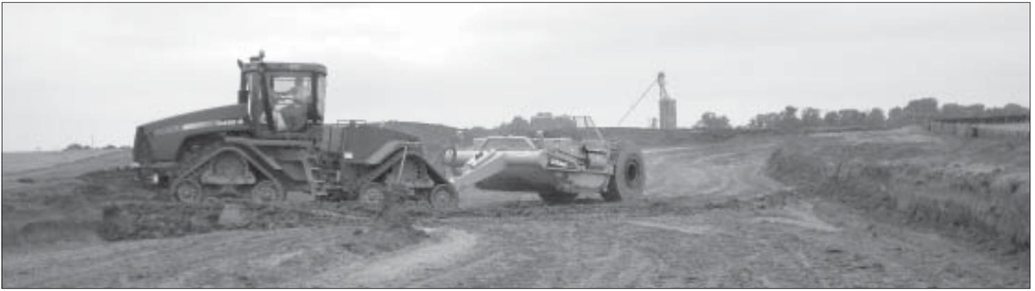
A crew from subcontractor Corrado American hogs out the top layer of dirt before starting the sanitary sewer line, which was installed 20 feet deep in the ground.
