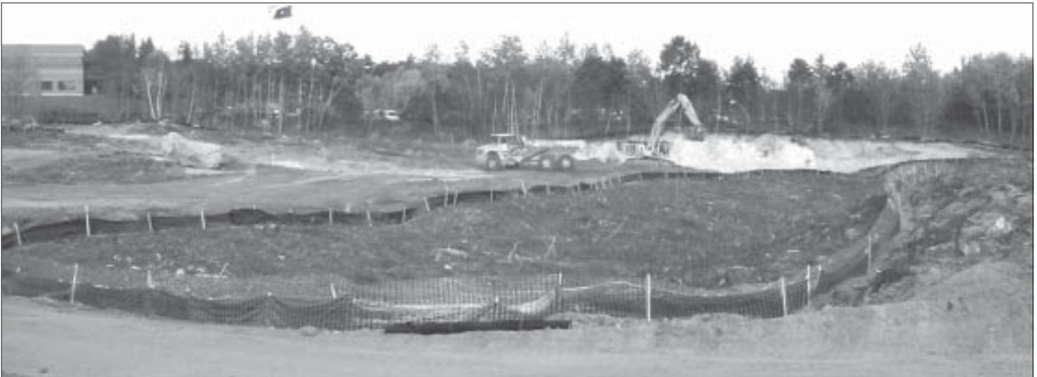
*Steve Renaud makes the cut from the future mitigated wetland area and adjacent pond (background). At center, a silt fence and construction fence has been installed around the existing wetland stream. This area must be protected until the mitigated area is completed. At bottom, a temporary crossing has been constructed as a haul road to remove the excavation.*
