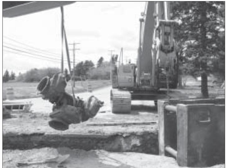
*A water service connection is lowered into the trench.*
