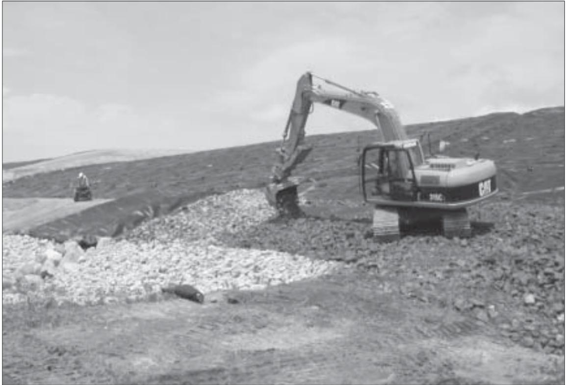
*Sargent crews place temporary cover at the Mt. Carberry landfill, which is covered with a temporary liner.*
