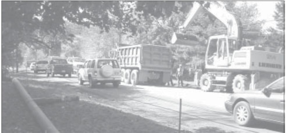
*Sargent crews dig a trench on the west side of Route 1 in Hampden. A temporary bypass force main (left) was placed on top of the ground on the east side of Route 1.*
