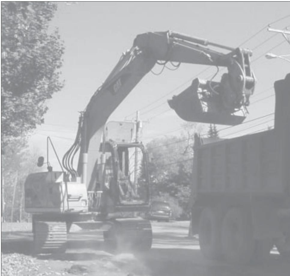
*Excavator removed the surface paving before digging the trench.*
