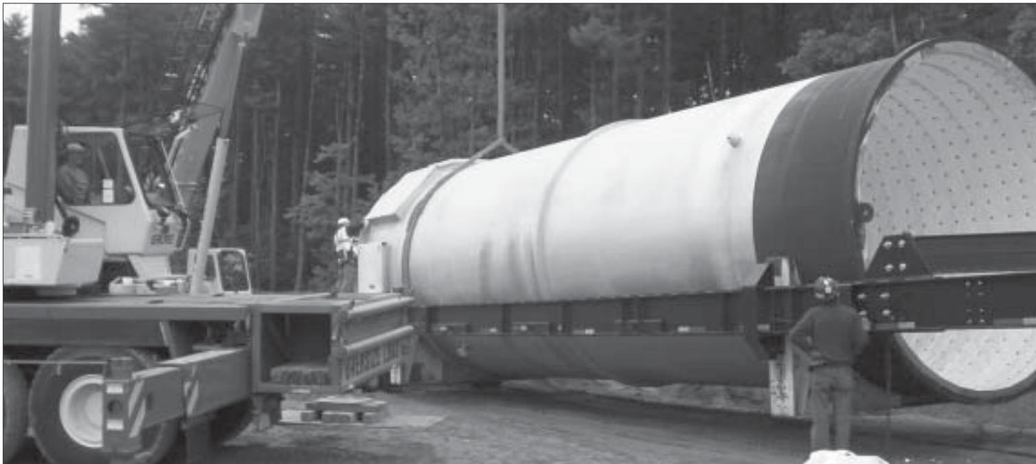
*Two cranes were needed to lift the silo off the flatbed and to set it on its pad.*
