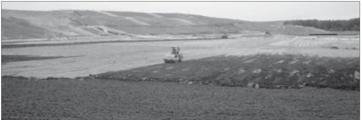
Foreman Roland Cloutier in the CAT CS-563E tries to keep up with the clay placement in preparation for upcoming rains. With crews placing clay at a record pace, the processing and compaction crew had to maintain a high performance level.
