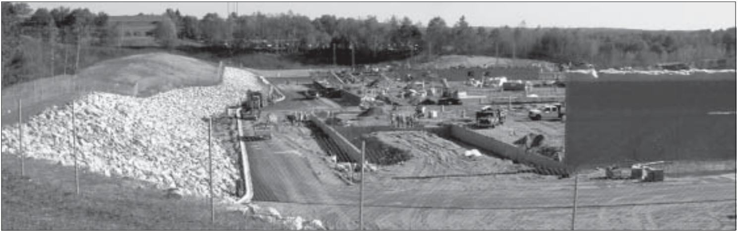
Four weeks into building construction, an excavator operated by John Dwinells excavates for interior column footings, while a rubber tired excavator operated by Mitch McLaughlin cleans up the building exterior.
