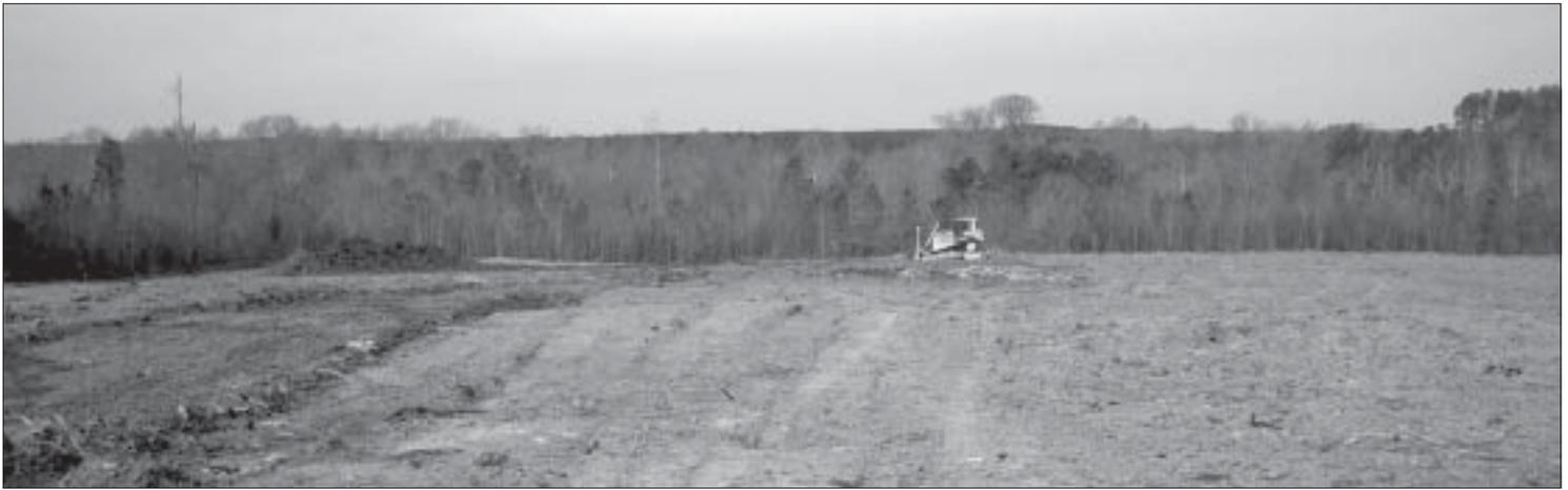
*Shannon Higgins uses the CAT D6R to push the overburden and stay ahead of the clay mining operation. Crews were forced to a new borrow area when the clay from the existing borrow area was used up.*
