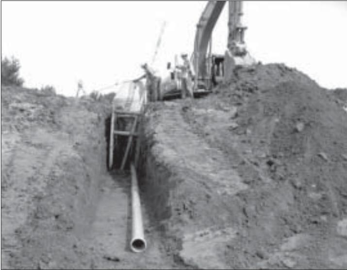
Sargent crews install 6" underdrain piping.
