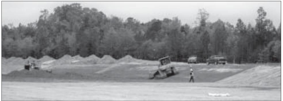
*Foreman Scott Bartlett checks the top of the clay elevations behind James Burnette in the CAT D6N to make sure the clay is ready for final certification before the liner crews arrive.*
