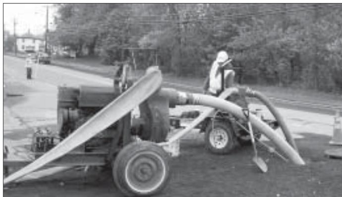
Sargent crews set up 6" and 4" bypass pumps due to high flows.
