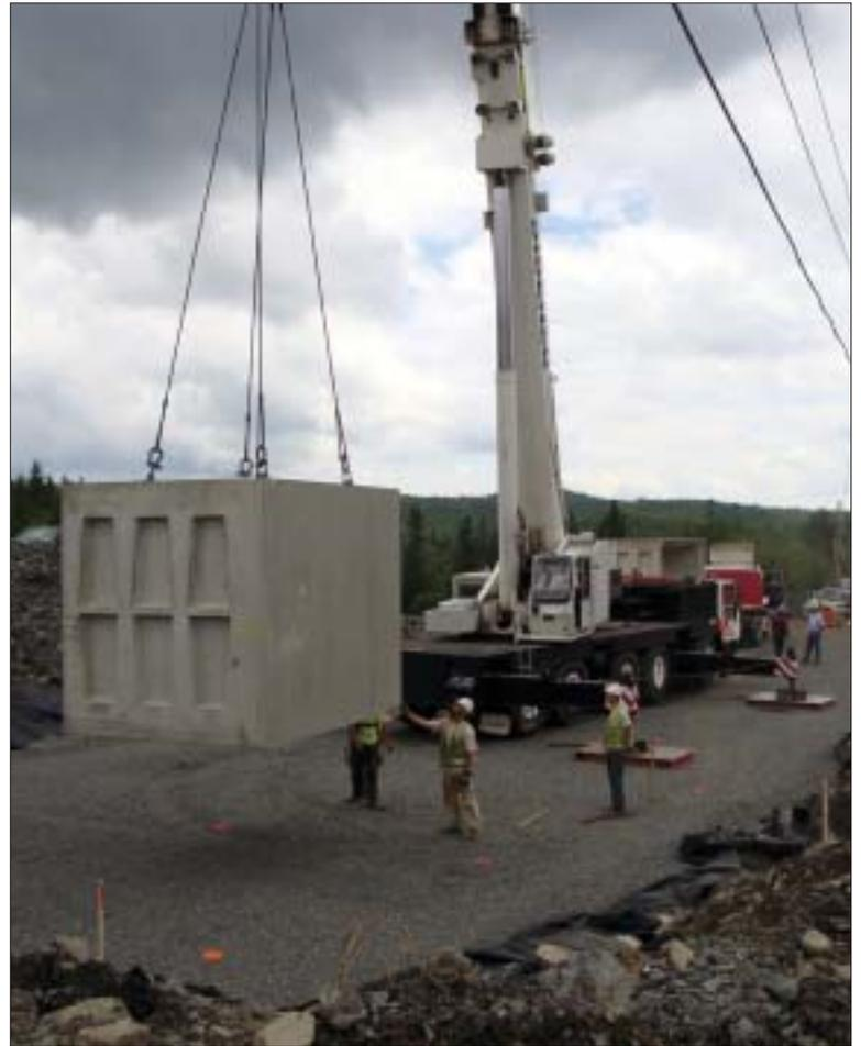
*Crane sets the first box culvert for the underground stormwater pond.*
