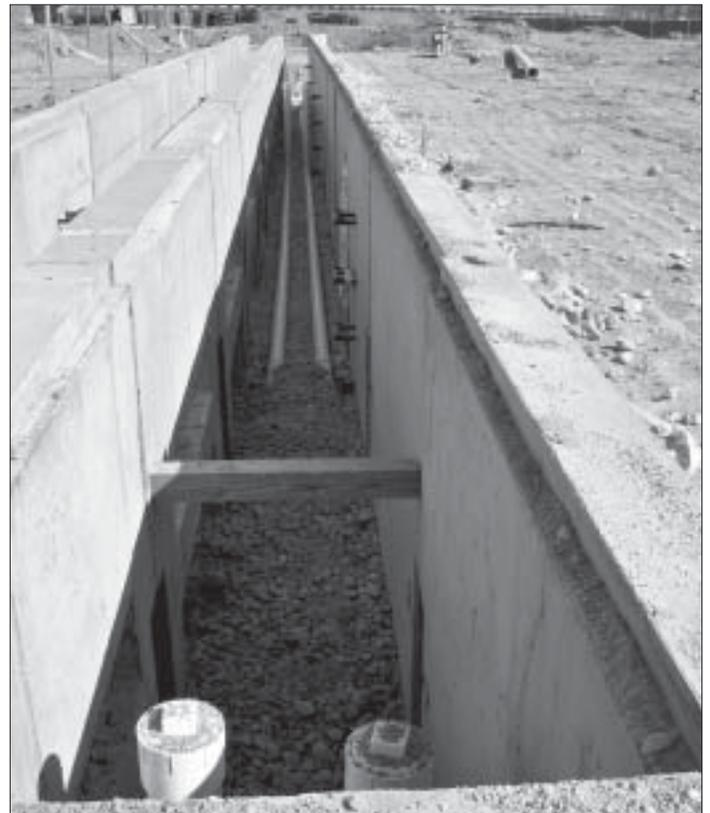
*Sargent crews install the sand filter stormwater device that leads to the underground detention system.*
