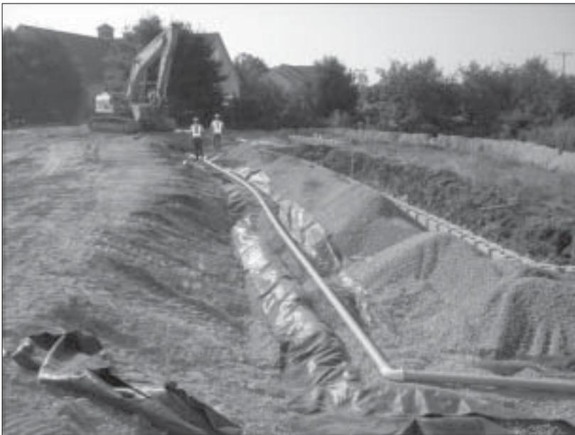
*Crews install the segmented retaining wall drainage system.*
