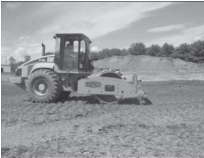
*Sargent crews use a CAT sheepfoot vibratory compactor on the stormwater detention pond.*
