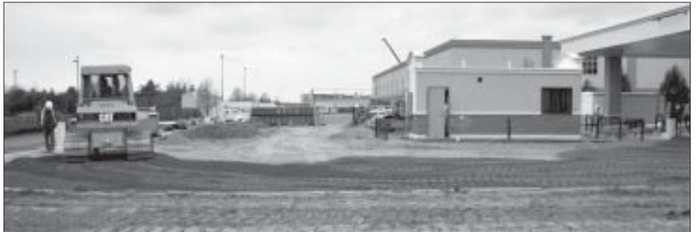
*Sargent crews spread stone in preparation for asphalt paving, as work continued on landscaping of the perimeter areas and completion of the kiosk and canopy areas.*
