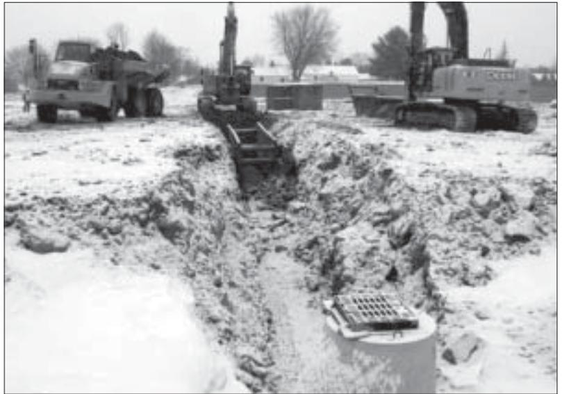
*Sargent crews install underdrain pipe in January 2009 as part of phase one.*
