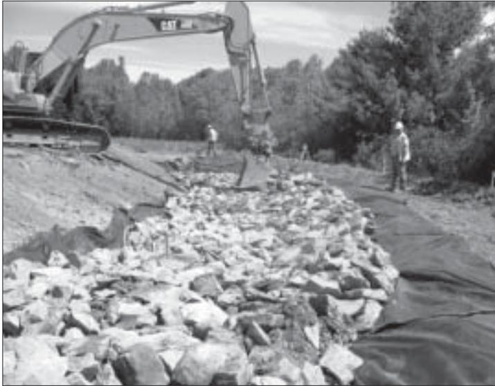
*A 30" layer of rip rap was placed in the outlet swale.*
