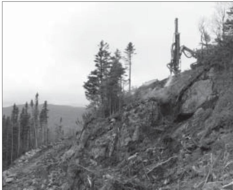
*A blasting crew from Maine Drilling & Blasting drills on “B” ridge. The access road is on the left.*
