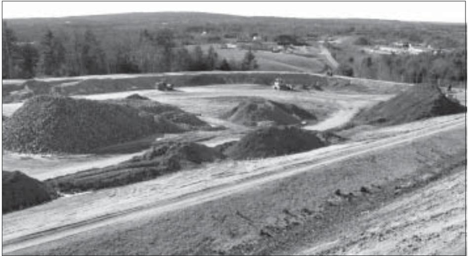
*Sargent crews work around stockpiles of processed rip rap and loam as they place common fill in the new cell during the fall of 2008. On a clear day, Mount Washington is visible in the background.*
