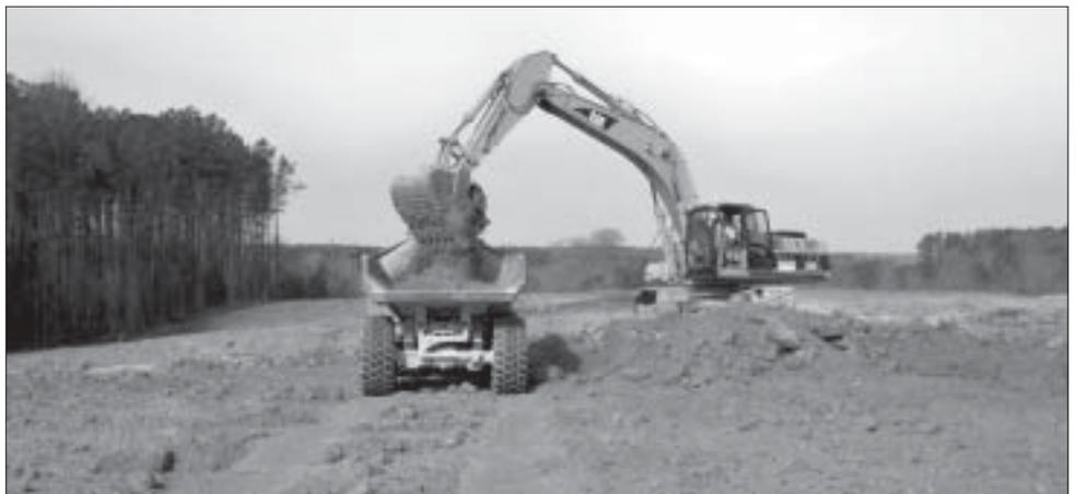
*Dave Walker in the CAT 330CL excavator loads clay from the borrow area into a CAT 735 truck. Dave and the foreman had to keep a close eye on the clay as the clay seams were not very thick.*
