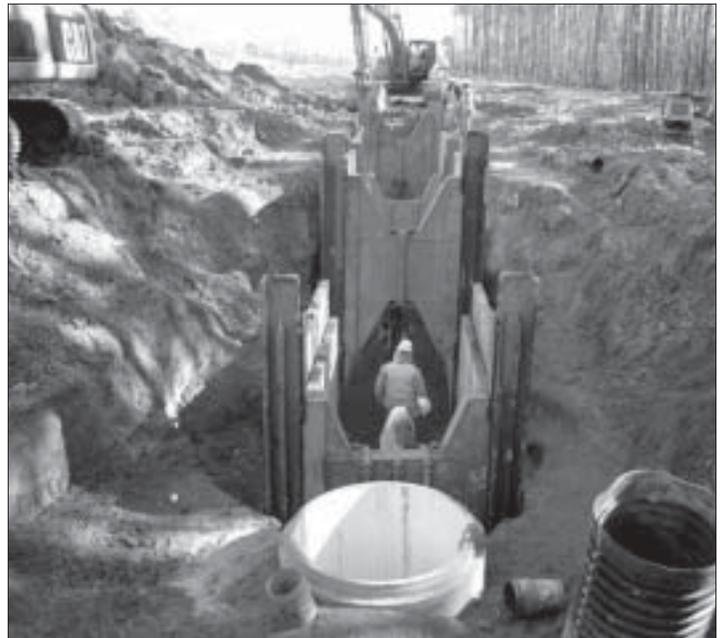
Sargent crew installs the gravity leachate main using a slide rail shoring system.
