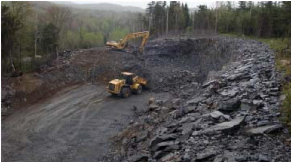
*CAT 325 excavator and 966 loader take a cut out of the south truck access road.*
