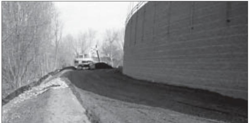
*A CAT 315 installs filter media in the bio-retention cell next to the retaining wall that Sargent constructed on the west side of the site.*
