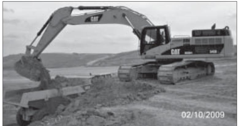
Bryan Smart in the CAT 345D L excavator loads a 4 Volvo A35D truck. The excavation crew moved 241,000 cubic yards on time and within budget.
