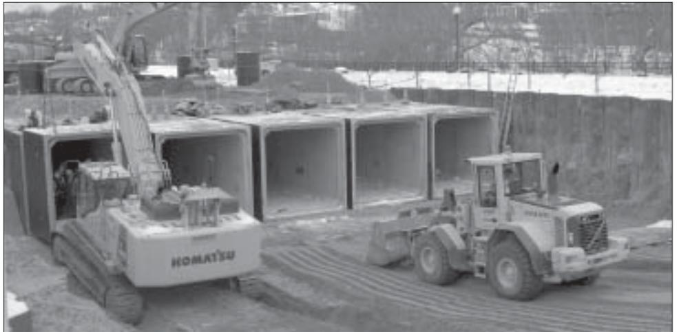
The Komatsu PC600 sets a box in place, while a front end loader grades the base of the site to ensure a level surface for the next row of boxes.
