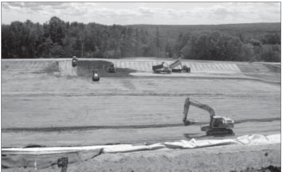
*Gerald Grindle uses a CAT D6N with GPS to place the secondary clay layer on the south berm and cell floor in June 2009. Ron Hall is on the sheepsfoot roller and Vicki Patchell is on the smooth drum roller. In the foreground, a 290 Volvo excavator operated by Steve Renaud exposes the liner tie-in.*
