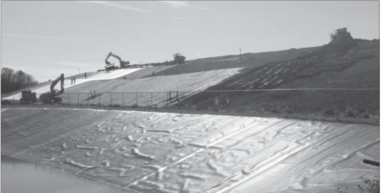
*The liner crew deploys the geosynthetic clay liner on the east slope of the Presque Isle municipal landfill.*
