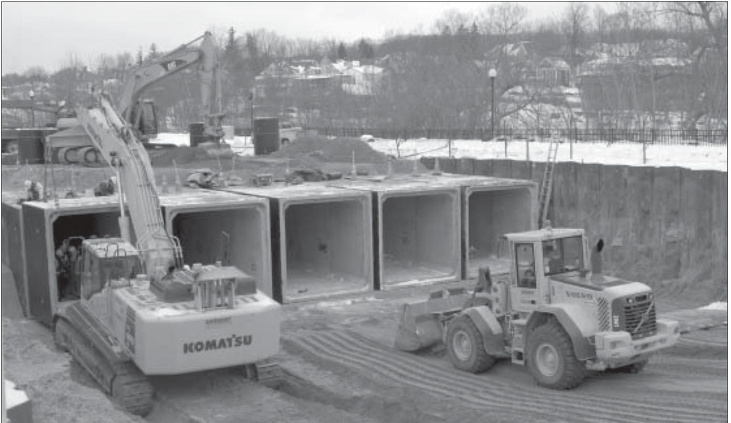
*The Komatsu PC600 sets a box in place, while a front end loader grades the base of the site to ensure a level surface for the next row of boxes.*
