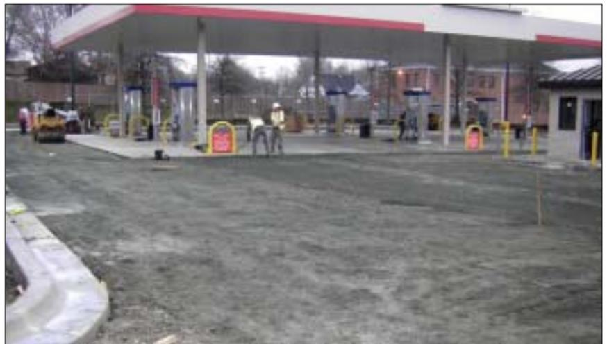
*The area around the fueling station was fine graded with a stone base and paved with asphalt.*
