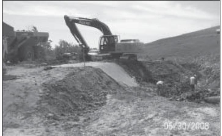
The crew shapes the clay and cleans around the gas header on the Phase VI Berm Project.
