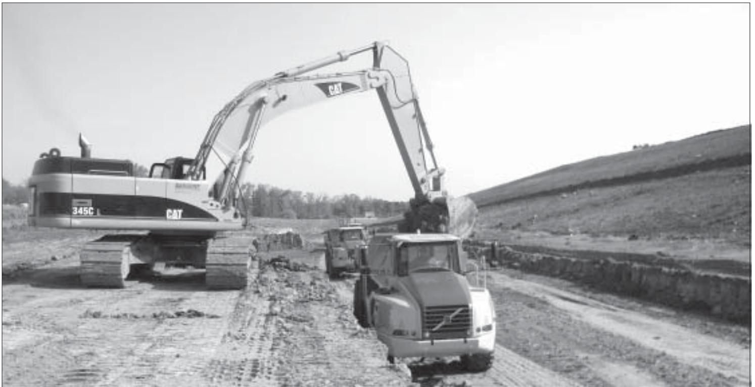
Excavator operator Bryan Smart loads excavated material into a rear dump at the Lorton Construction Debris Landfill in Lorton, VA. A total of 300,000 cubic yards of material is being excavated to construct the new 12-acre cell at Lorton.
