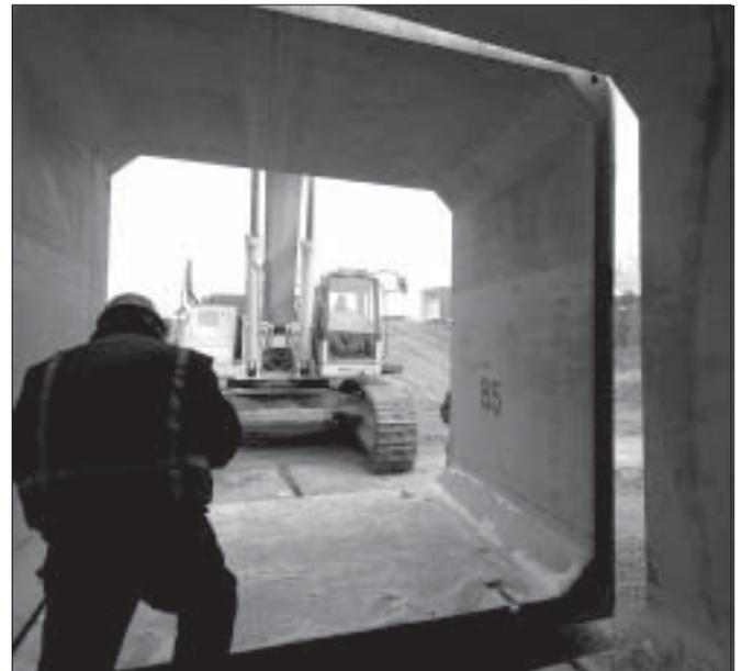
*A total of 250 pre-cast concrete chambers were used to create the 1.3 million gallon storage facility.*
