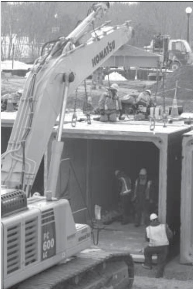
*Sargent Corporation based its bid on using its Komatsu PC600 excavator to set the pre-cast concrete boxes, or chambers, in place (above and below) instead of renting a crane. The PC600 was operated by Steve Renaud.*
