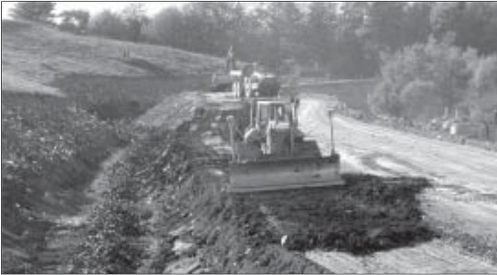
Sargent crews place and shape clay on the Phase VI Berm Project at the Pine Tree Landfill in Hampden. Brian Loisel is on the Cat D6N, Ken Thurlow on a John Deere 270, and Everett Spaulding is on a Komatsu 35 ton haul truck.
