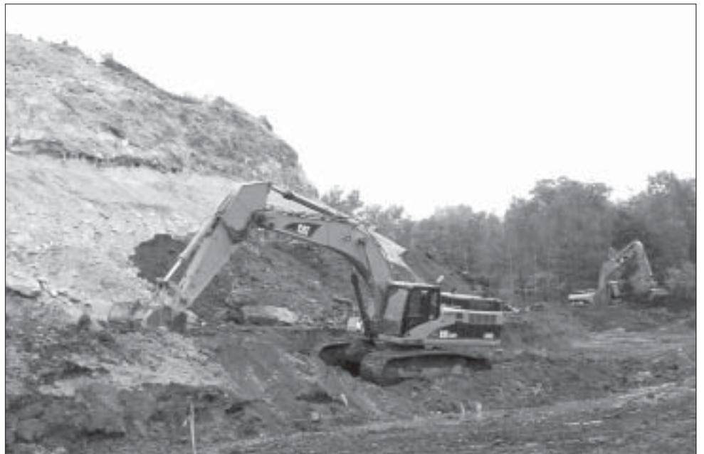
*Kempton Bradbury, operating the Cat 345C in the foreground, prepares to install the 6" toe drain around the leachate pond, as Mike Brant builds leachate pond berms in the background.*
