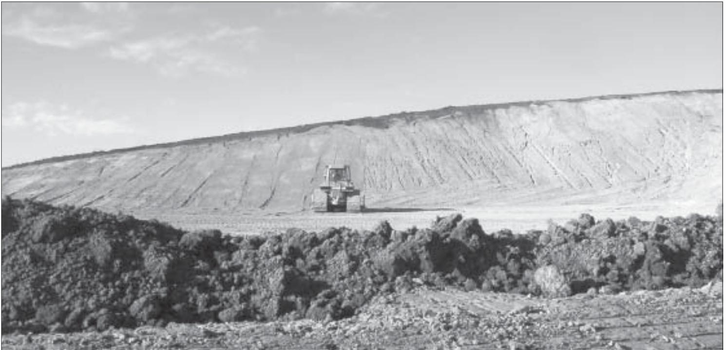
*Danny Whipple, operating a Cat D6N dozer, grades the CKD pile at the Dragon Cement landfill to prepare it for the clay cover and then for the short paper fiber/loam mixture.*
