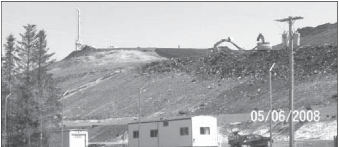
Recovery Drilling drills for gas wells on the Secure II landfill, while a John Deere 270 operated by Ken Thurlow and a Liebherr 904 operated by Mike Hamlin install gas piping as part of the Closure Project.
