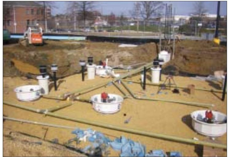
*The crew backfills the tank pit with pea gravel.*
