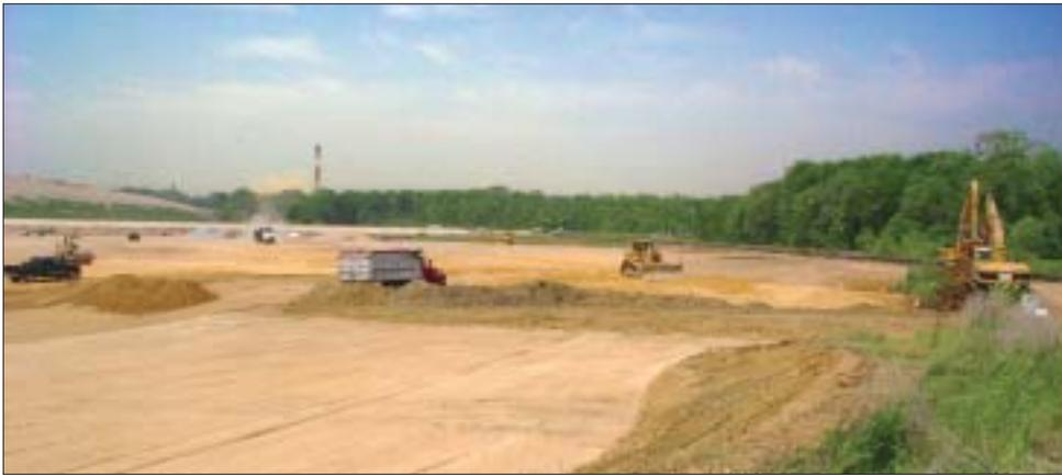
Imported borrow is placed on most of the site. Foreman Justin Porter directs the unloading, placement and compaction activity, as operator Joe Garrett runs the D6N dozer while Ricardo Diaz operates the roller.
