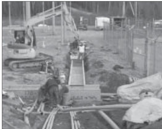
*Above and below: Sargent crews install precast electrical duct bank at the Bangor-Hydro Orrington substation.*
