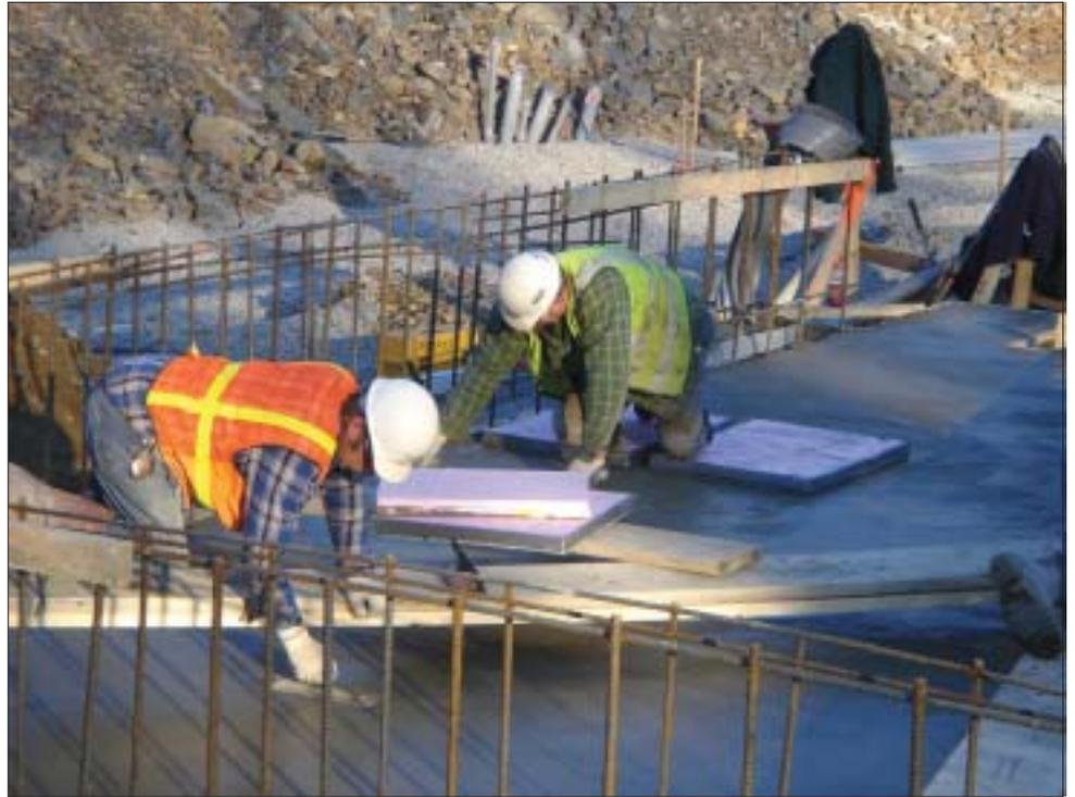
*Peter Heath and Fred Clements finish the concrete work for the base slab for the hopper building foundation at the Ogunquit transfer station.*
