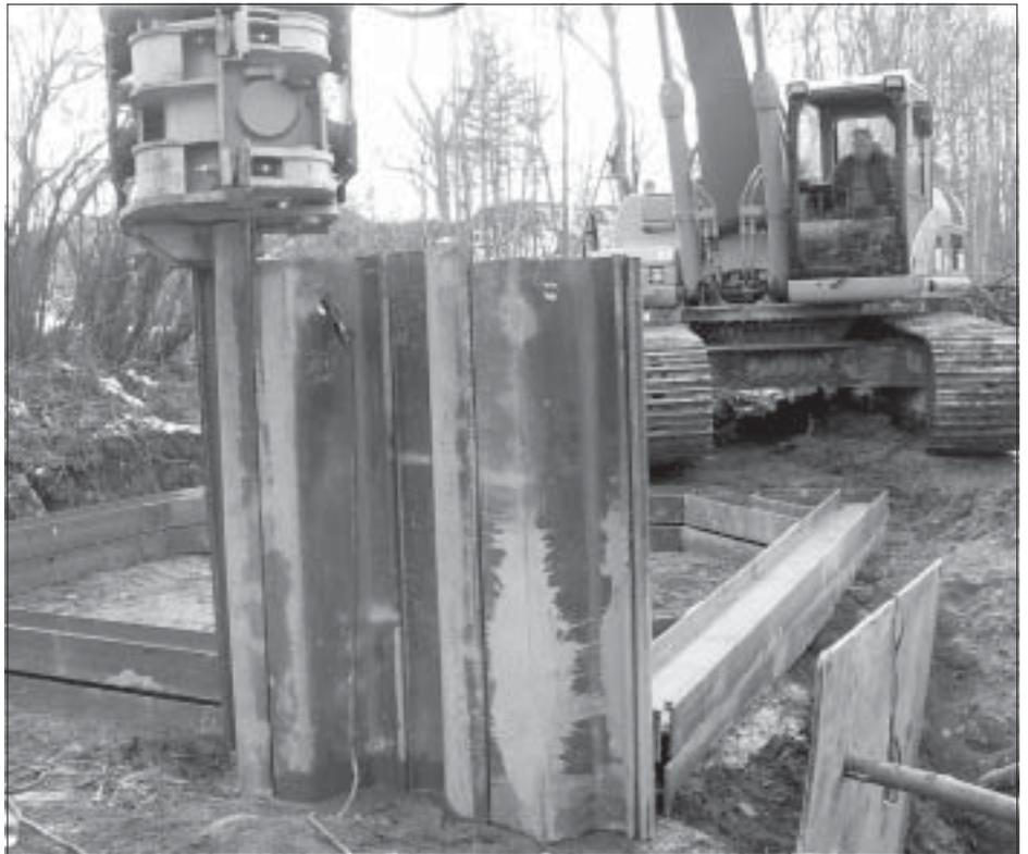
*Sargent's new Hercules sonic-powered sheet pile driver.*
