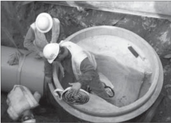
Sargent crew installs a 30" sewer line into one of the 5' diameter manholes on the Augusta Whitney Brook Project
