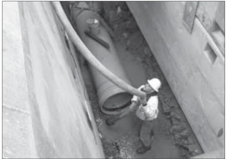
Shawn Newton dewatering one of the many 16' plus deep trenches to install the 30" sewer line on the Augusta Whitney Brook Project.
